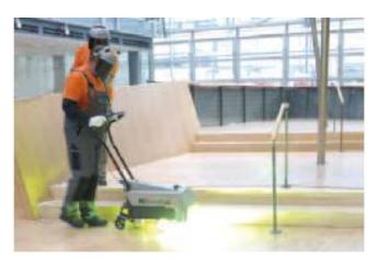
LOBA – the surface specialist for parquet and hardwood floors – is bringing a revolutionary, UV- curing floor-finish system to the market: LOBACURE WS Rush A.T. is ready for practical application. With this system freshly fitted or refurbished hardwood floors can reach full hardness and usability in less than half the normal time. The finishing process, which can easily take five days using conventional
